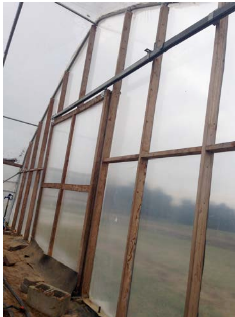
Wood framed endwalls require some construction knowledge.
