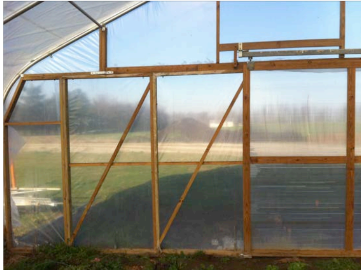
All of these wooden panels are removable, opening up the end of the tunnel considerably.
