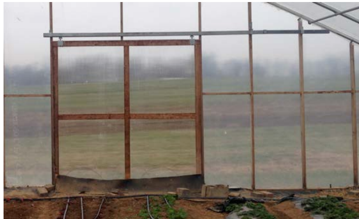
A moderately sized equipment door designed for use with a walk behind tractor.
