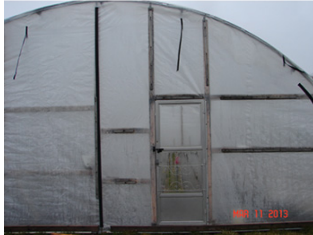
An example of a repurposed screen door serving as an access door Source: ipm.illinois.com
